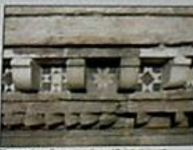
The cornice after restoration with intact mortar.
